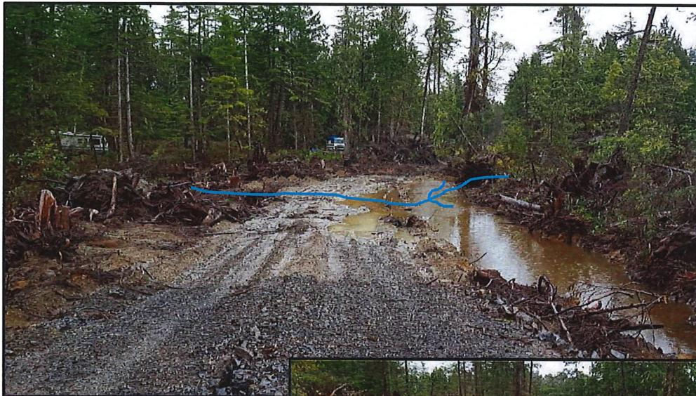
Photo 7: View on opposite side of road alignment in campground area. Clearing went through lower part of drainage.
